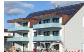
9,5 kWp Photovoltaik-Mieter-Strom Hallbergmoos, 2015
