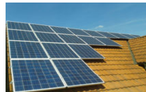
9,4 kWp Photovoltaik-Mieter-Strom Wolfersdorf, 2015
