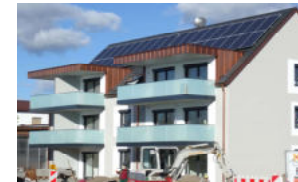
9,5 kWp Photovoltaik-Mieter-Strom Hallbergmoos, 2015
